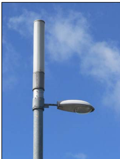
This mast on Embankment Road has been designed to look like a street lamp.
