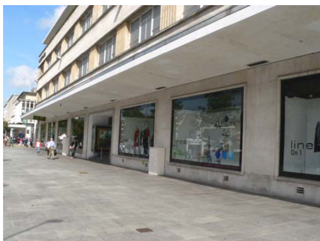
City Centre shop front showing stall riser, windows and framing and solid canopy.
